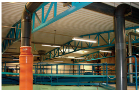
Sewage water treatment plant
